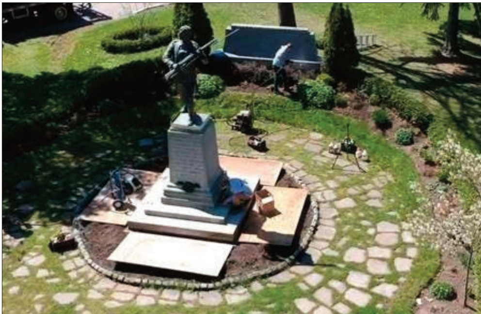
Cenotaph work being done. Summer 2021.
