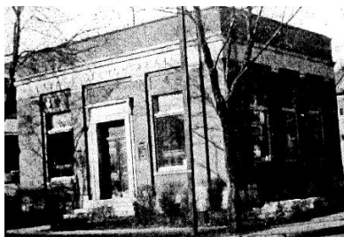
The Bank of Montreal at 101 avenue Westminster North was built in 1930
